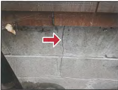
Small foundation crack, right side
