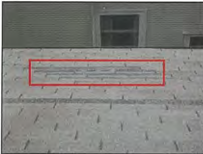
Worn, missing shingles
