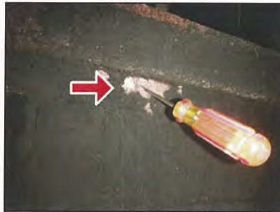
Deteriorated bricks in firebox
