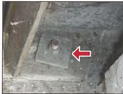
Anchor with bearing plate
