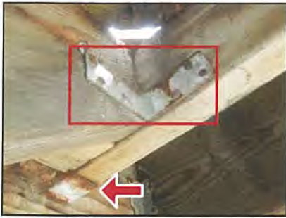
Corroding deck/stair hardware
