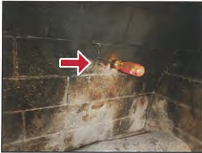
Soft firebox mortar
