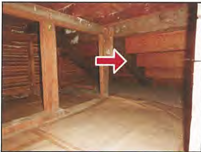
Exposed stair underside
