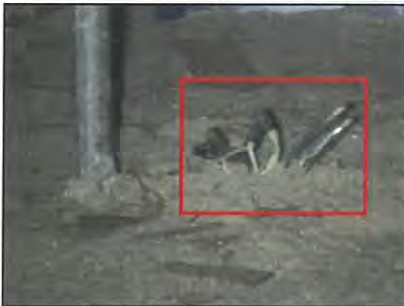
"Running splices" in attic
