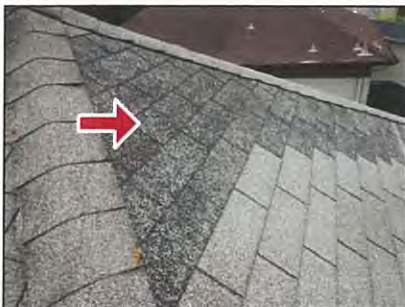
Extensive granule loss
