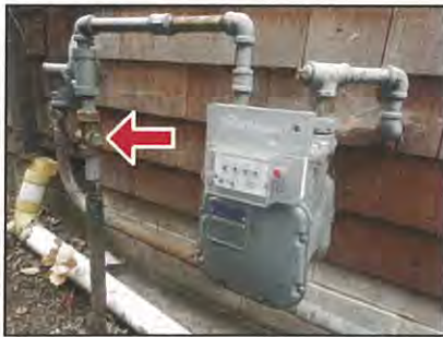
Gas meter & main shut-off valve
