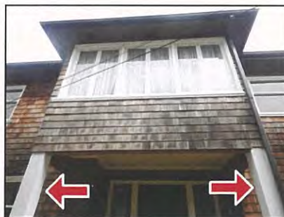
Potentially weak supports
