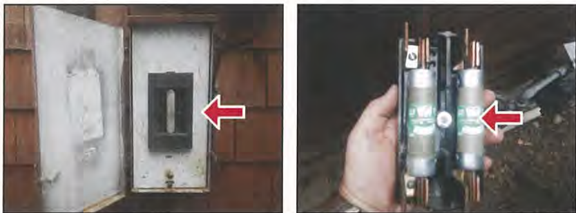
Main electrical disconnect
