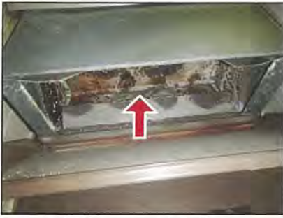
Rusted draft diverter
