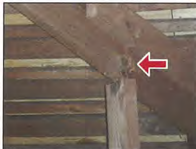
Crack at knot in rafter
