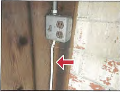
Exposed Romex cabling
