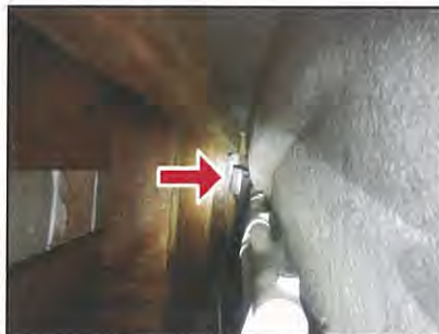
Inaccessible GFCI &amp; pump
