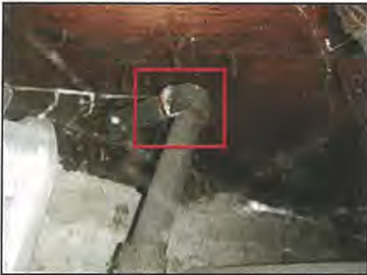
Corroding piping in crawlspace
