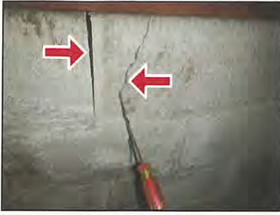
Cracks in basement wall
