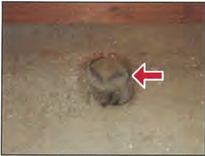
Outdated anchor, no bearing plate
