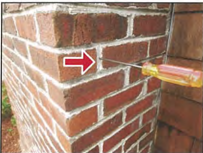
Soft, deteriorated chimney mortar
