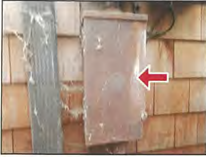
Rusted main panel enclosure
