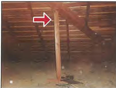
Post supporting cracked rafter
