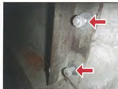
Loose nuts at angle irons
