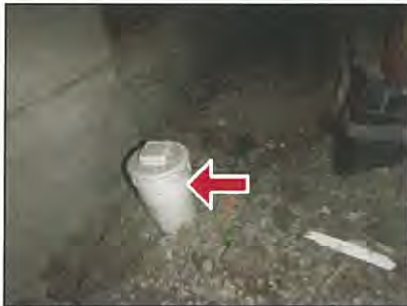
Drainage cleanout
