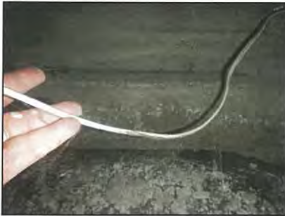
Unsecured wiring in crawlspace
