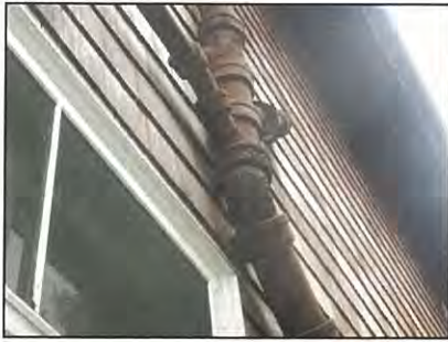
Corroded drain piping
