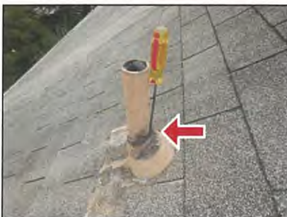
Deteriorated vent seal
